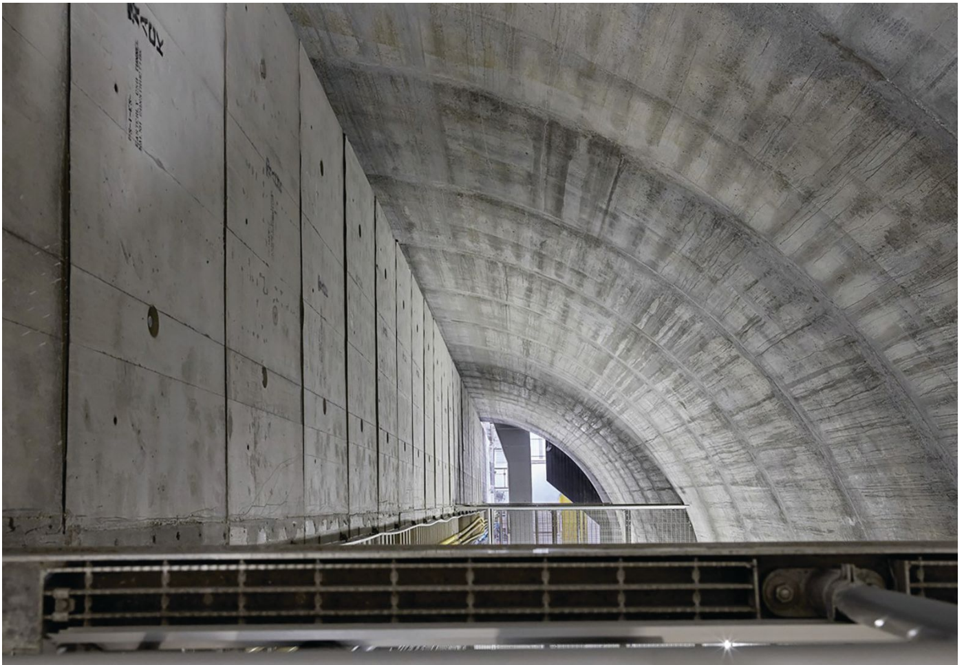
In some communities where space and the resources allow, enormous stormwater diversion tunnels are constructed to capture and retain excess stormwater during heavy rain events.
